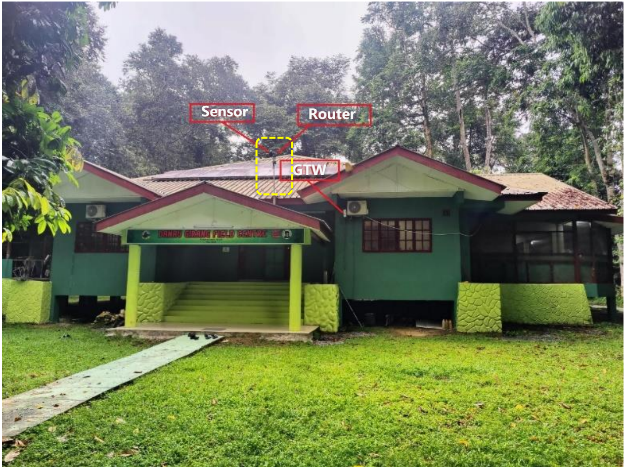
Figure 2.1. Photos of installation location 1, the main building with annotations to show locations for the sensor, router, and gateway. Figure 2.2 below shows a closeup of the sensor and router, in the yellow dashed square.
