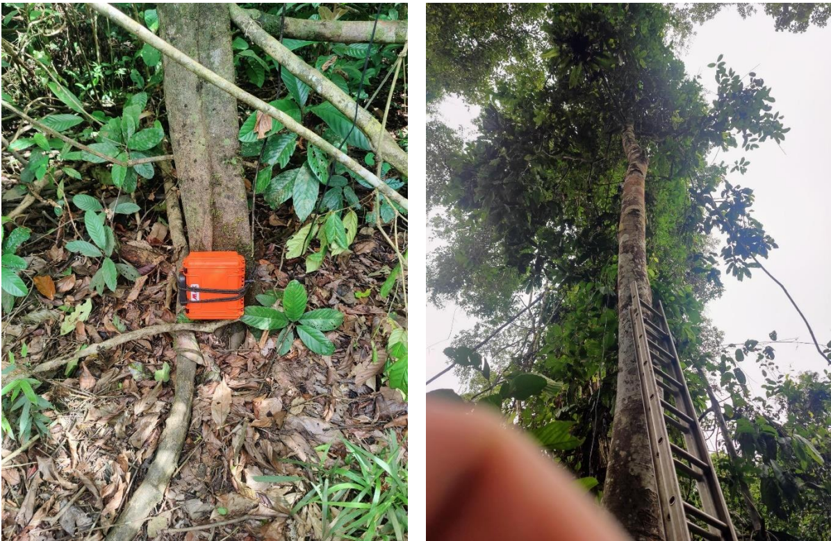
Figure 3. Photographs showing the deployment of the battery pack (left) and the router (right) for deployment location 2.
