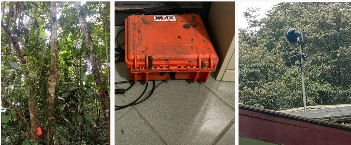
(From Left to Right) both the rechargeable battery pack and the sensor attached to a tree, rechargeable battery pack, sensor installed on top of the DGFC main building roof
